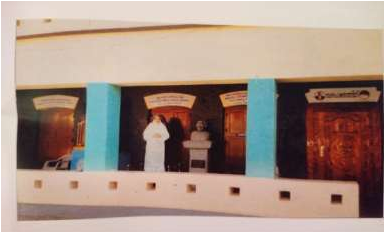
The Convent Constructed by Msgr. Joseph Kuzhinjalil
